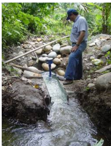
Figure 4– Vietnamese 200 W low-head pico-hydro 'propeller' unit installed in Ecuador
