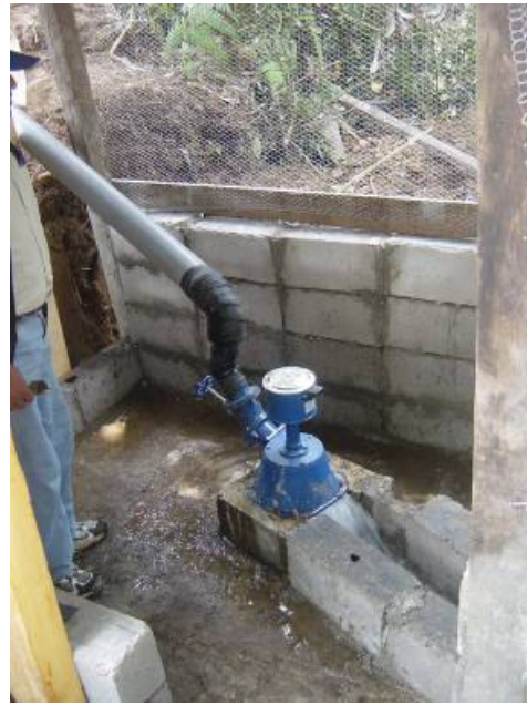
Figure 3 – Vietnamese 200 W medium-head pico-hydro 'turgo' unit in Ecuador
