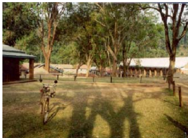
A front view of the Kisiizi Hospital Complex (Photo from Kisiizi Hospital website).
