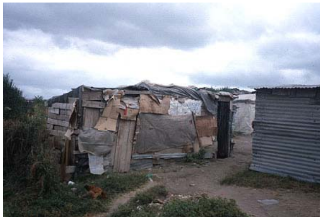
Construction using a variety of scrap materials in Kasweto , lack of awareness on appropriate low cost building materials has contributed to inability of the poor to upgrade their housing . Credit: Theo Schilderman.
