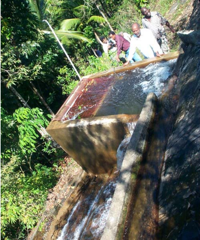
An example of a penstock at the source of the hydro intake. In Hettikanda and Handunella, this was built by the community
