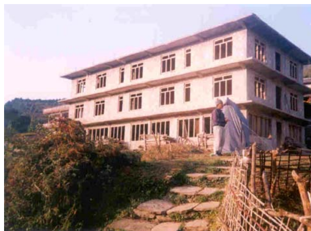
New hotel under construction in Ghandruk
