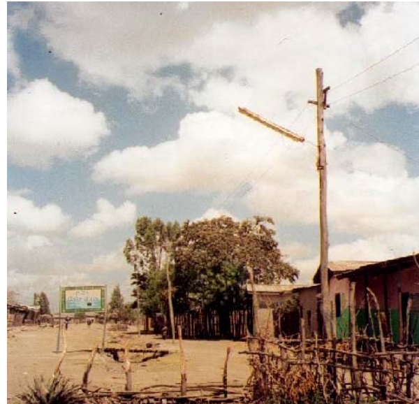
Streetlighting and transmission lines in Bonosha
