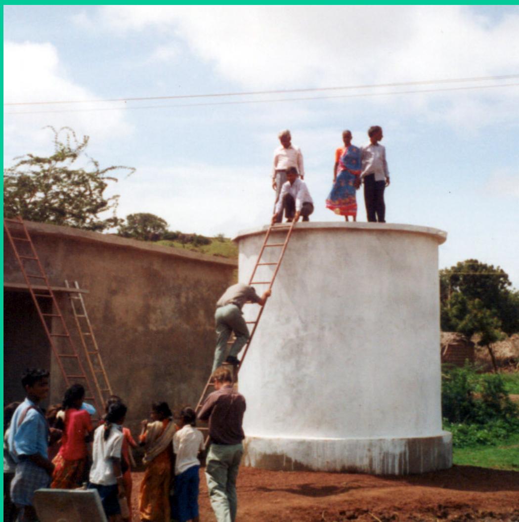
Reinforced-concrete grain bin at Mizapur (13-tonne capacity)
