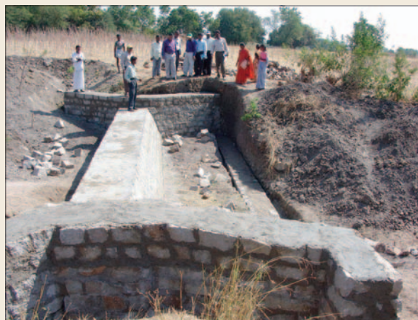
Check dam in Chowderpalli
