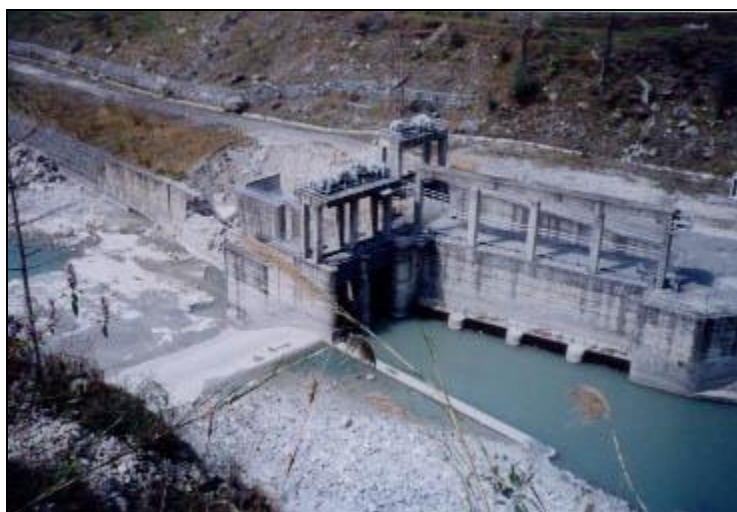
Figure 6. The intake of the Modi Khola Hydroelectric Project, March 04
