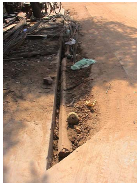
Figure 3.10 Side drain damage at Puok
