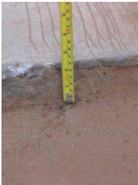
Figure 3.9 Maximum shoulder erosion
