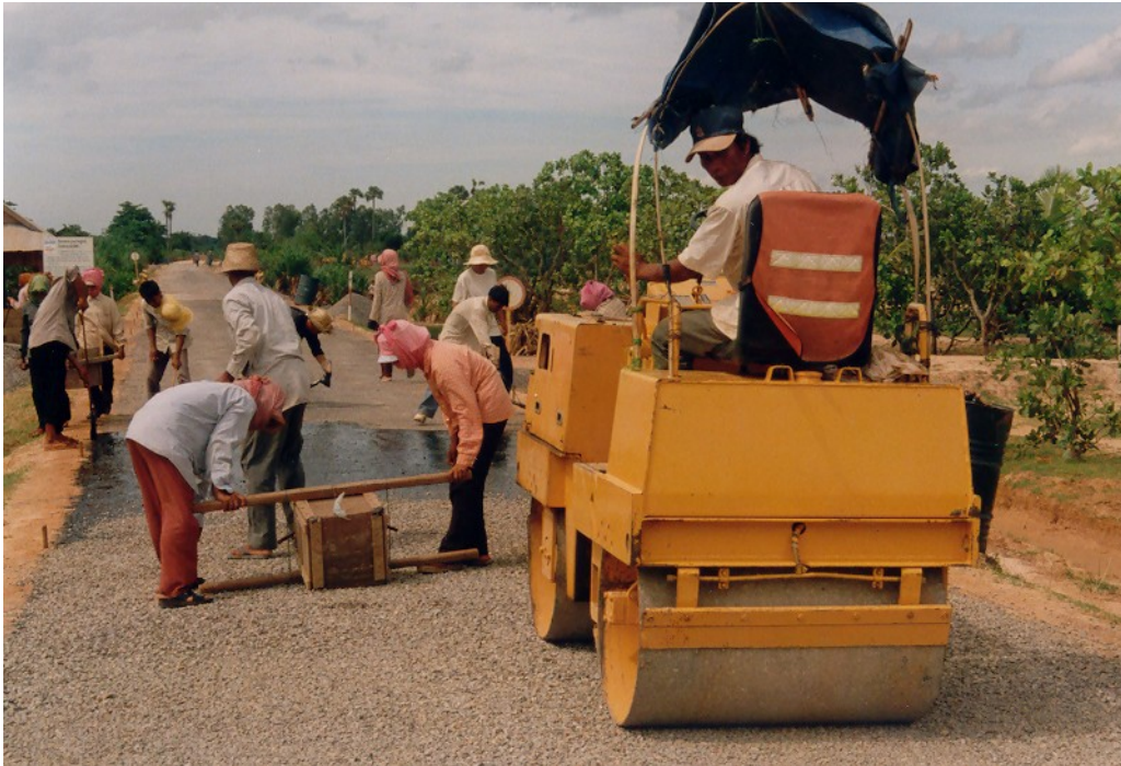
Figure 1.2 Puok Trials construction works
