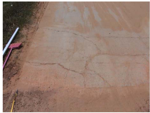
Figure 3.8 Cracking on final slab, ILO paving
