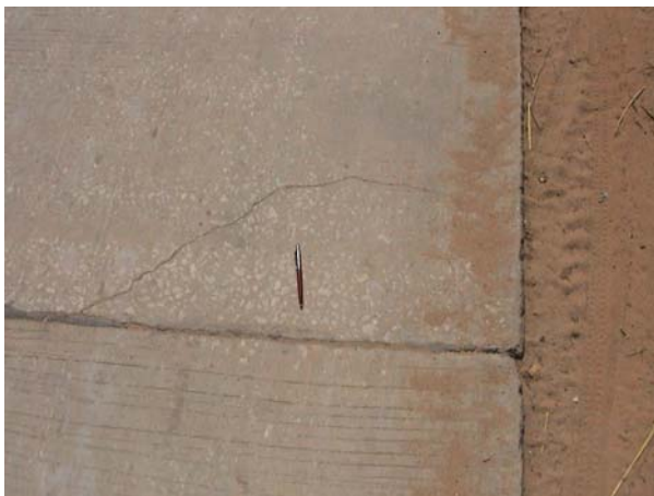
Figure 3.7 Single slab crack
