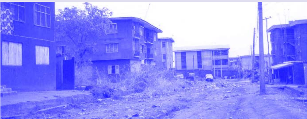
Apartment blocks in Achara, informal subdivision, Enugu
