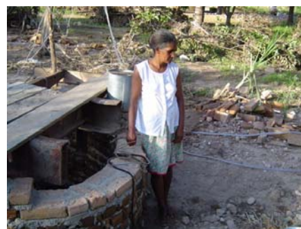
Dug Well used for Irrigation and Domestic Supply
