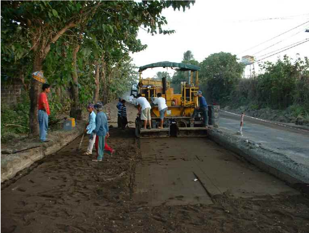
Plate 2 Construction of the stabilized sub-base
