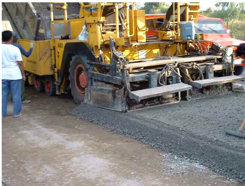
Plate 4 Construction of the crushed stone base
