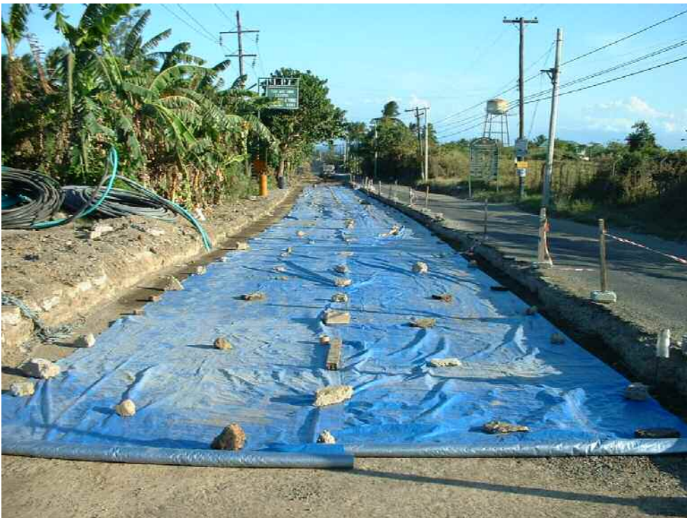
Plate 3 Curing the stabilized sub-base
