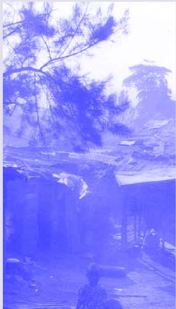
Rudimentary structures that serve as drinking joint in Kamwokya
