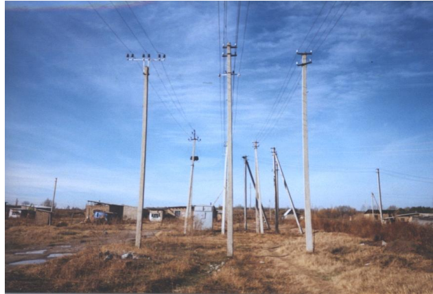
New transformer cabin in Ak Bosogo
