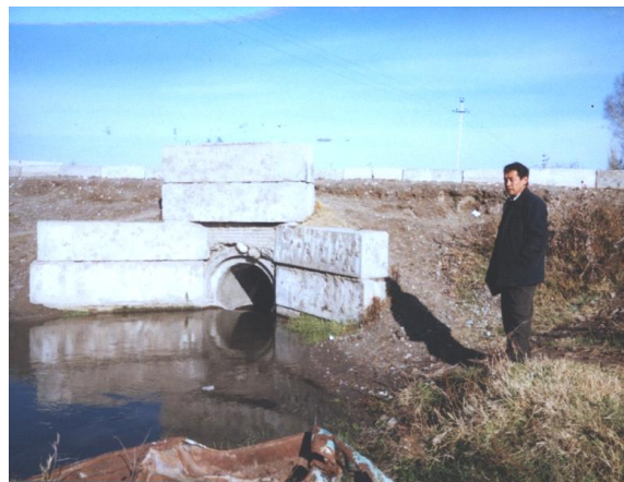
Local NGOs provide capacity building to enable communities to engage with government structures for the provision of a range of infrastructure services, such as roads.
