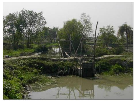
Plate 3 Control of water through bunds, sluices and canals at Jorria. Seen here is a sluice gate supplying water to the waterbody from the main water channel (Source: R. Arthur).
