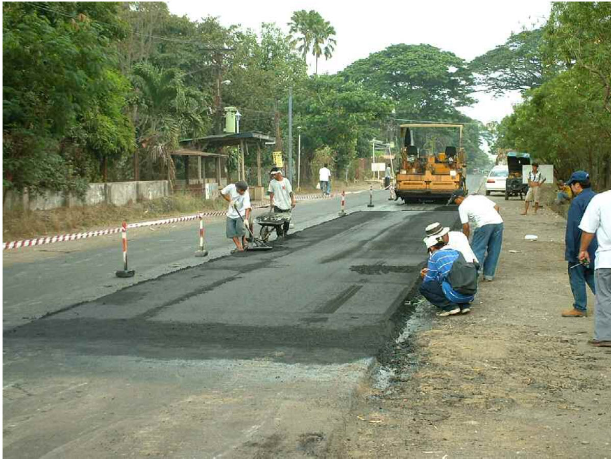
Plate 1 Compaction trial: hot rolled asphalt
