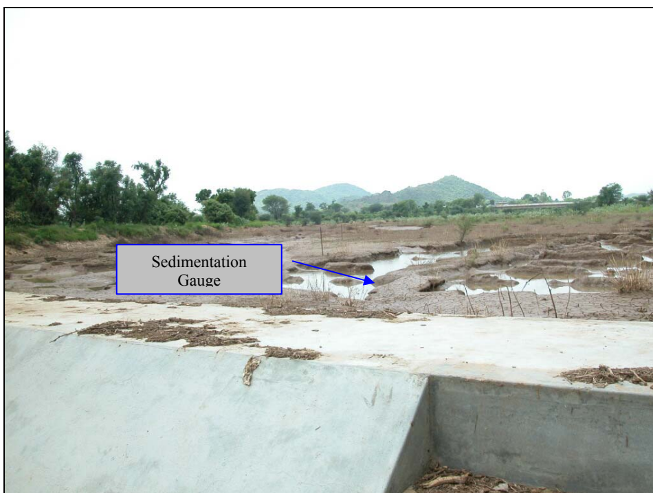
Plate 11. Sedimentation Gauge fixed in Bhanawas check dam
