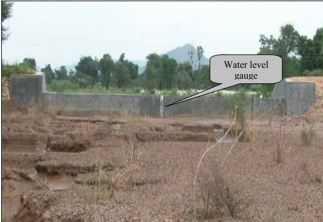
Plate 9. Water level Gauge in the check dam, Bhanawas
