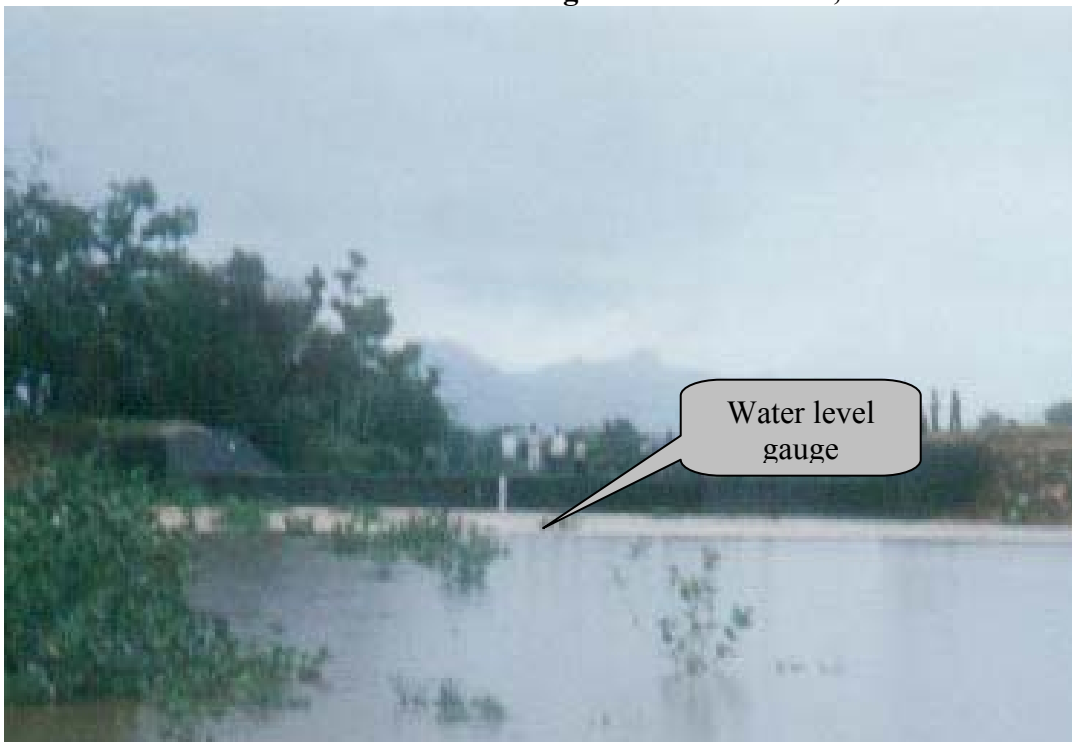
Plate 10. Check dam filled with water and the level gauge, Bhanawas village
