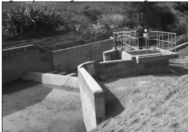
Fig 4. Improved irrigation intake in Usangu
