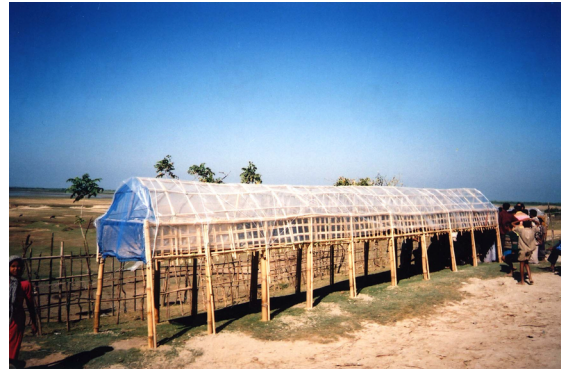
Figure 2. Low cost locally made solar drier
