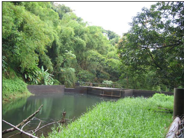
Figure 2 – an example of one of the many small dams from which water is abstracted by NAWASA
