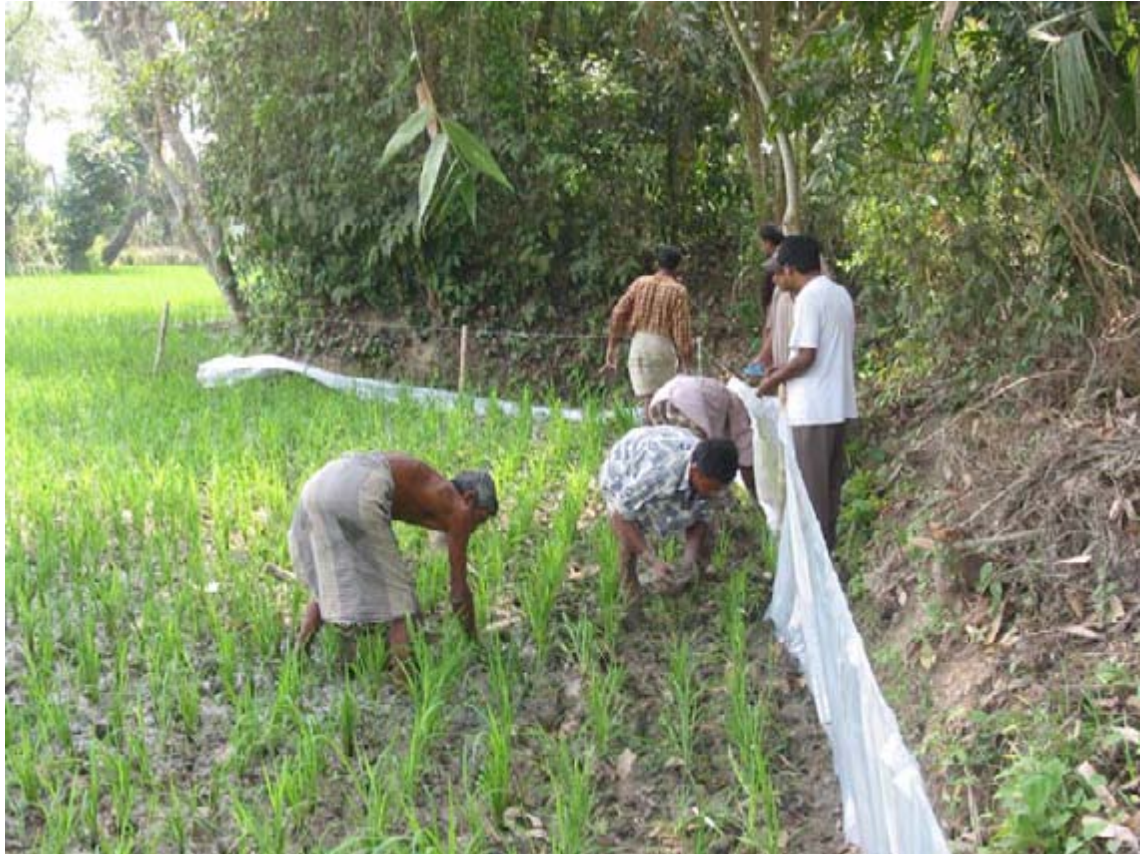
Figure 65. Photograph of LTBS under construction
