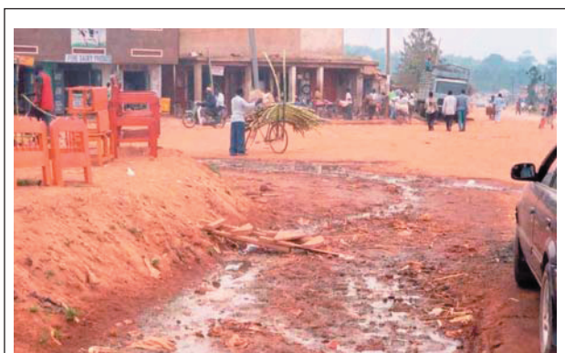
Photograph 1. Surface runoff needs managing
