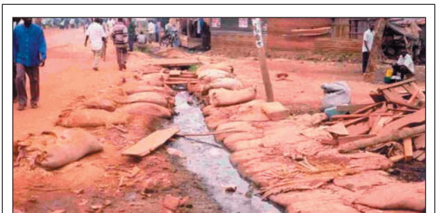
Photograph 10. Using sand bags to divert surface flows
