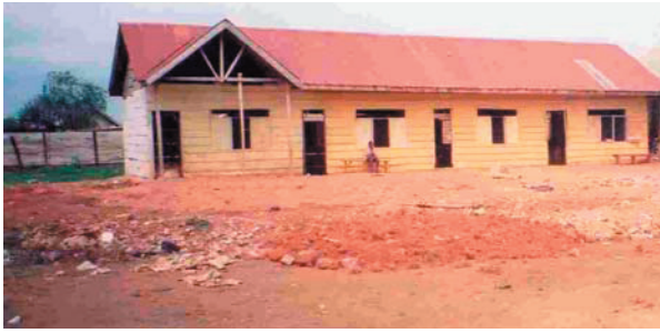
Photograph 11. Raising the ground level to avoid flooding
