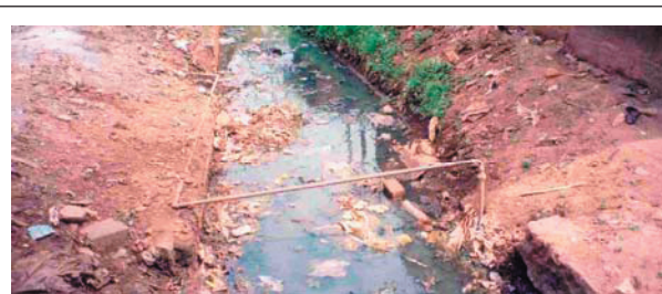
Photograph 2. Water pipes crossing drains are vulnerable
