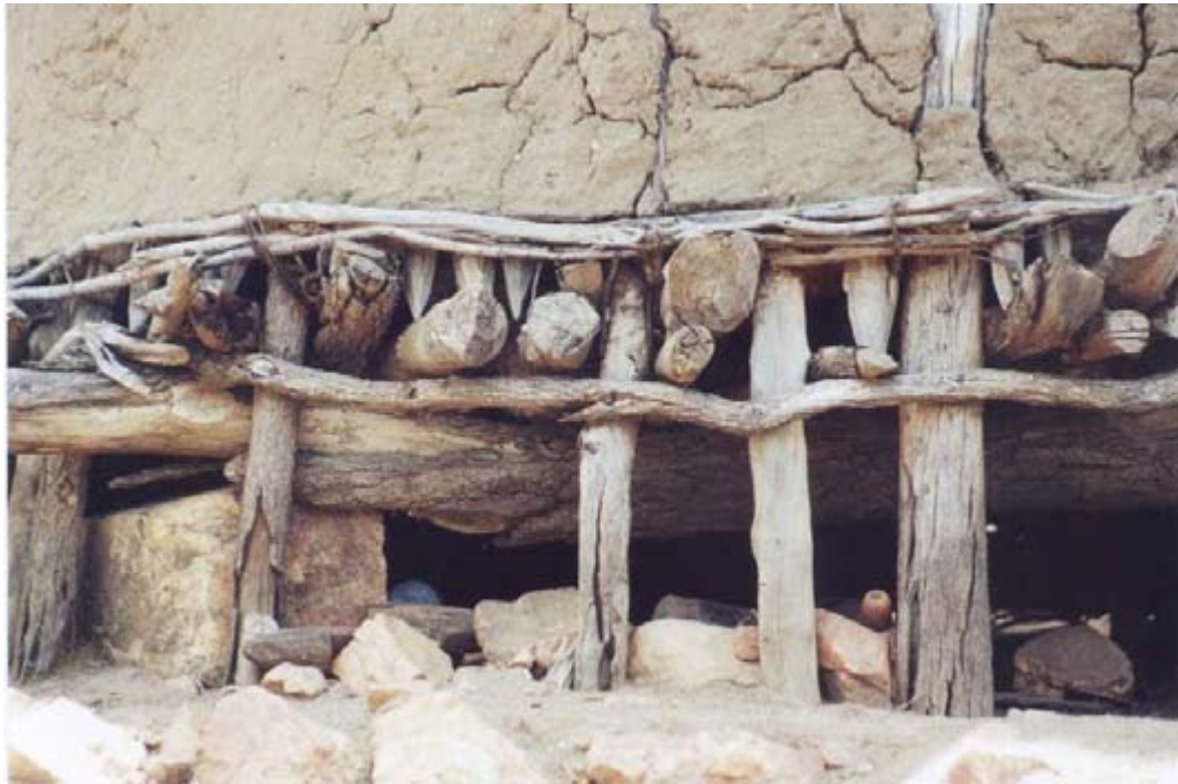
Plate 1.1. Rodent damage to food storage; entry holes in the base of a dulu granary
