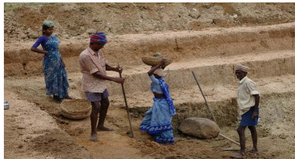
Farm pond under construction near Pujenahalli Tank
