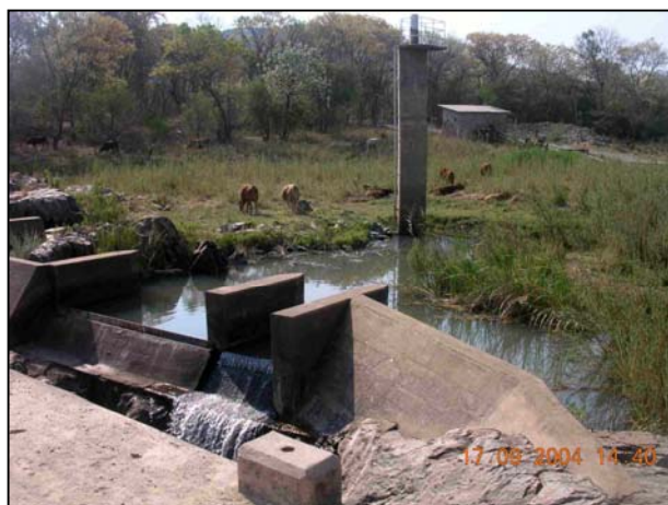
Fig. 2. Thuli River at Freda Mine.
