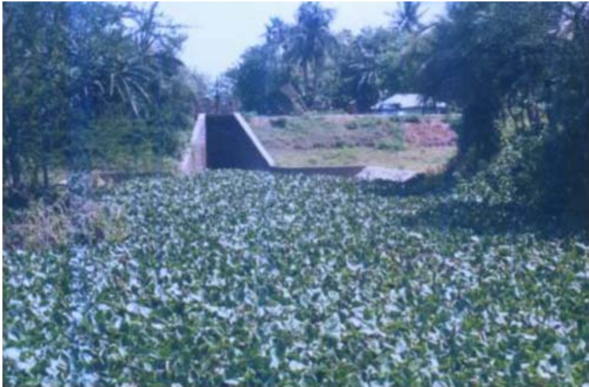
Goakhola Sluice from khal side, dry season 2003-04
