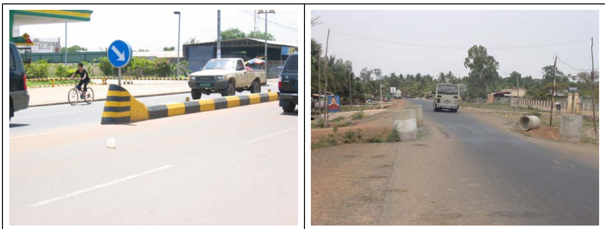
Figure 12 Solid concrete structures present considerable hazards to errant vehicles. The start of the concrete median barrier should be chamfered up gradually from road level, despite the consequential need to replace the 'keep right' arrow sign more frequently. Right hand photo shows road narrowing due to culvert protected by concrete pipe sections: a hazard particularly at night.
