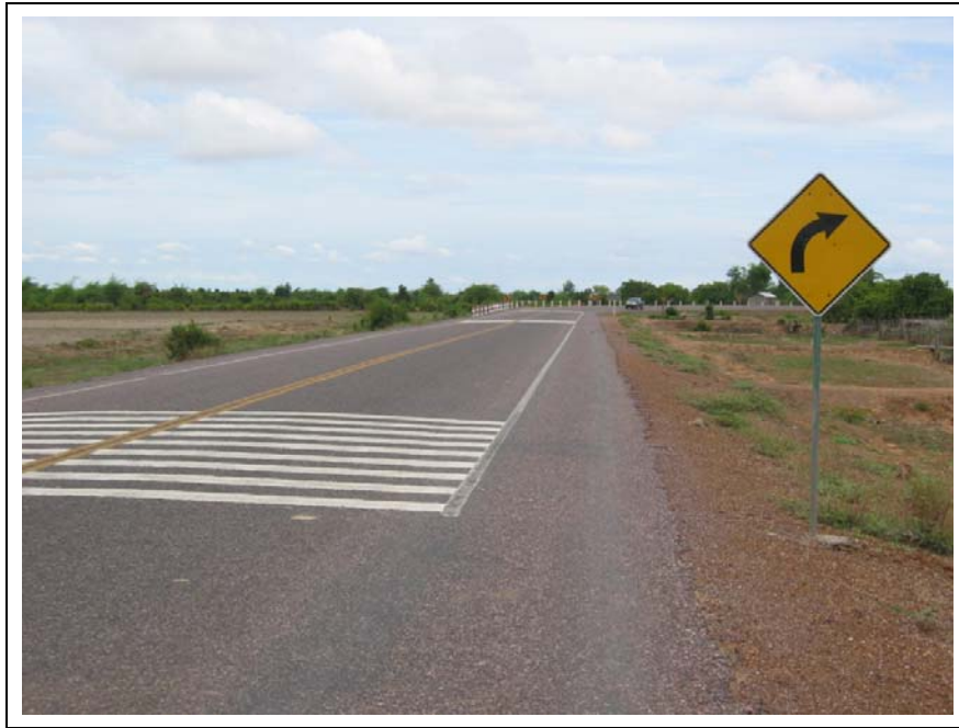
Figure 6 Sharp 90° bend after long straight section, initially unmarked – should have been noticed in an audit. Good warning devices (signs, jiggle bars, chevrons) subsequently installed.
