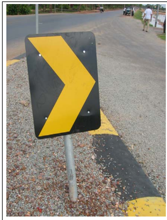
Figure 9 Chevron sign: a very helpful and cost-effective warning device on bends, though much better if (diamond-grade) reflective material used.
