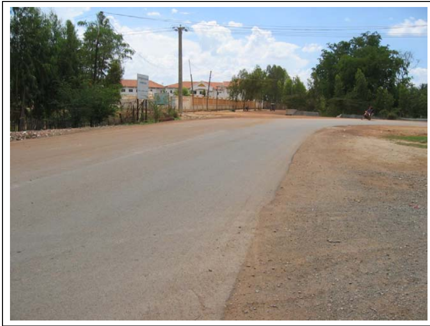
Figure 8 Blackspot identified by Traffic Police on toll road in Phnom Penh: a sharp right bend after long straight section with no signs or marking. Driver sightline is down avenue of trees straight ahead – probably a greater hazard at night-time.
