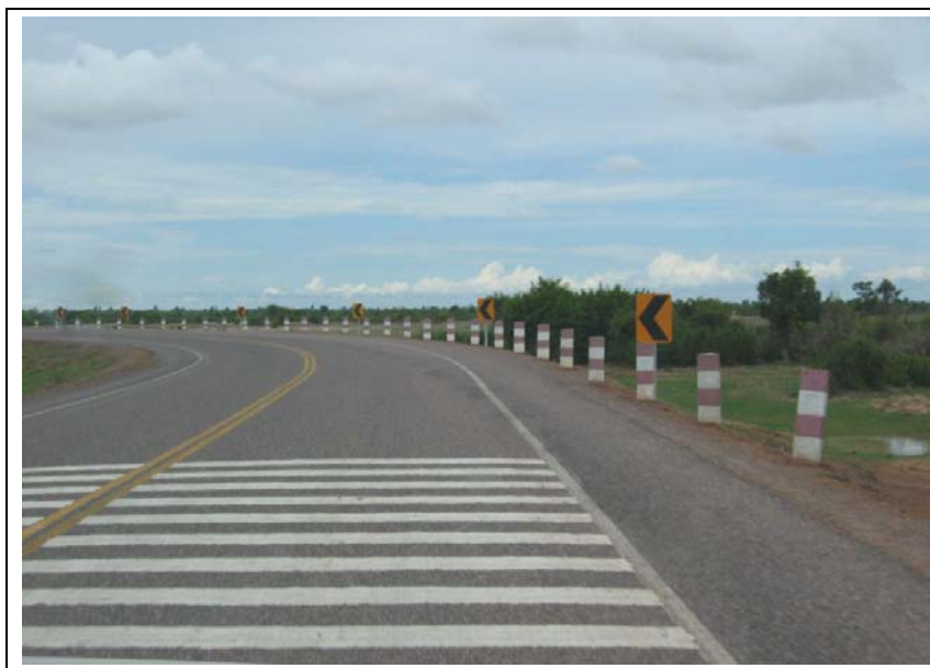
Figure 15 Section on NH6 with separate marked cycle/pedestrian lane, and good warning for sharp bend: including rumble strips, edge delineator posts (though more 'forgiving', collapsible posts would be preferable) and chevron boards.
