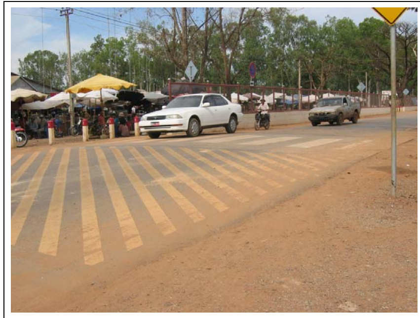
Figure 10 Owing to complaints from drivers through village, the original flat-topped humps with steep sided ramps were extended to long humps as shown above, which can be driven over comfortably at 60km/h. Preferred standard would be 3.7m long, 100 to 120mm height and segment of a circle in cross section. This shape is still suitable for raised zebra crossings.
