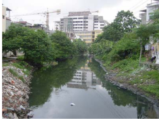
Figure 4 The stormwater drainage system in Hanoi is heavily polluted
