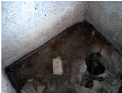
Photo taken by students of dirty toilet in a Zambian primary school
