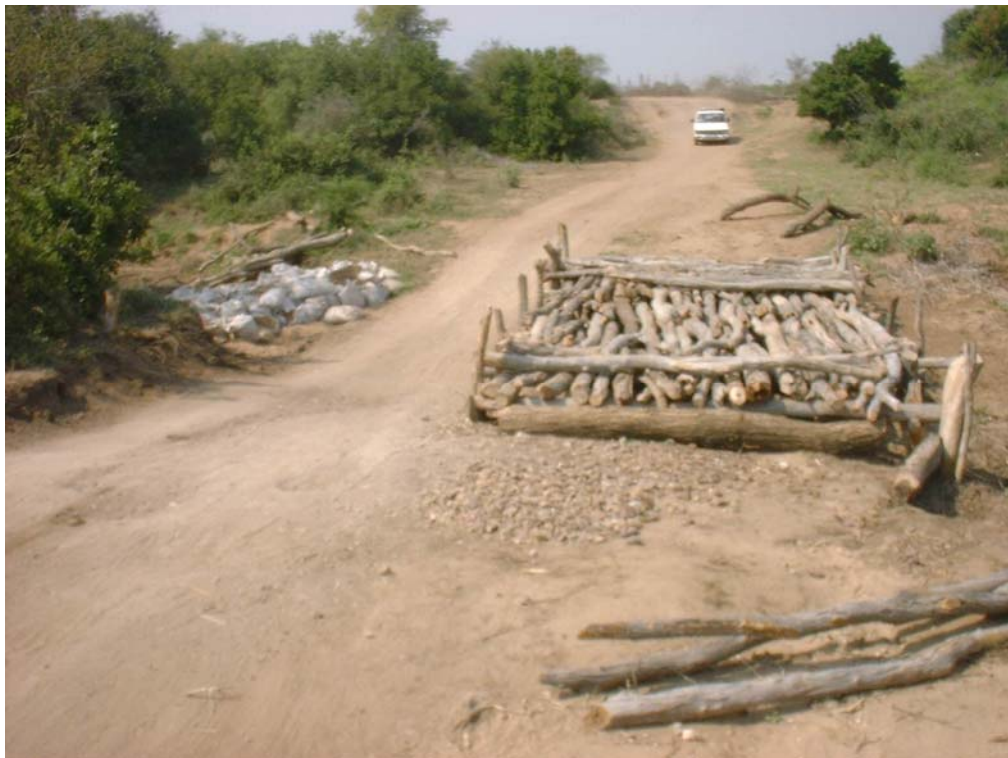
Figure 2.11 Access road showing bridge deck construction.
