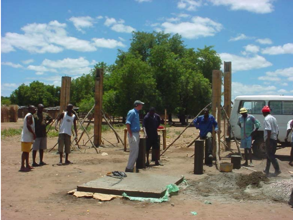
Figure 5.3 Construction in progress
