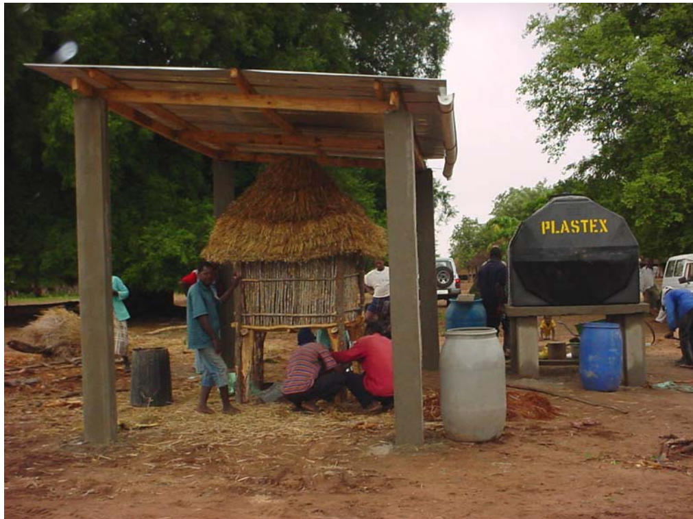
Figure 5.4 Rainfall harvesting facility and seed store nearing completion
