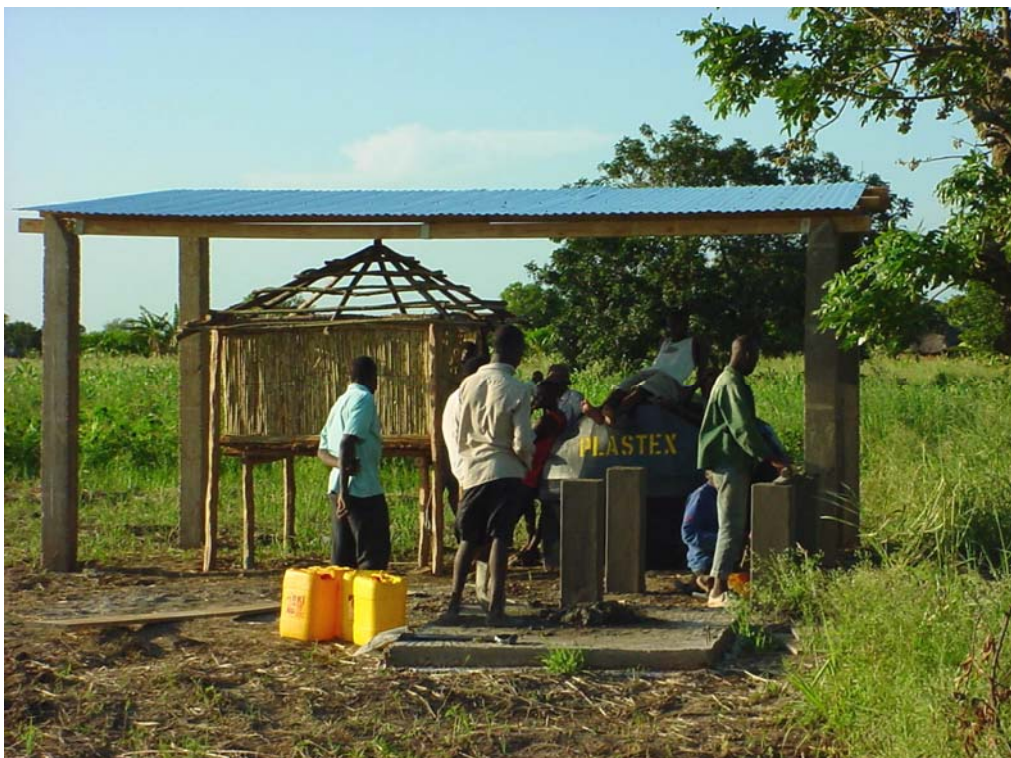
Figure 5.4 Construction of water tank support
