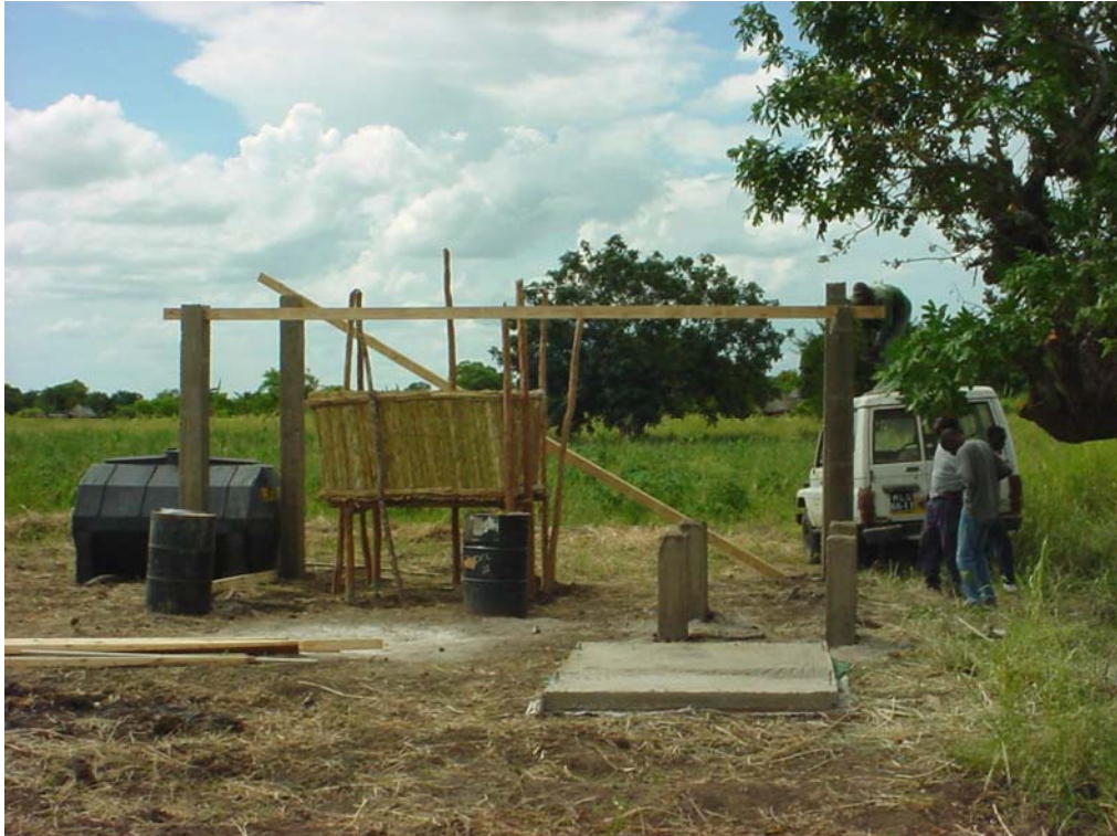
Figure 5.3 General view of construction
