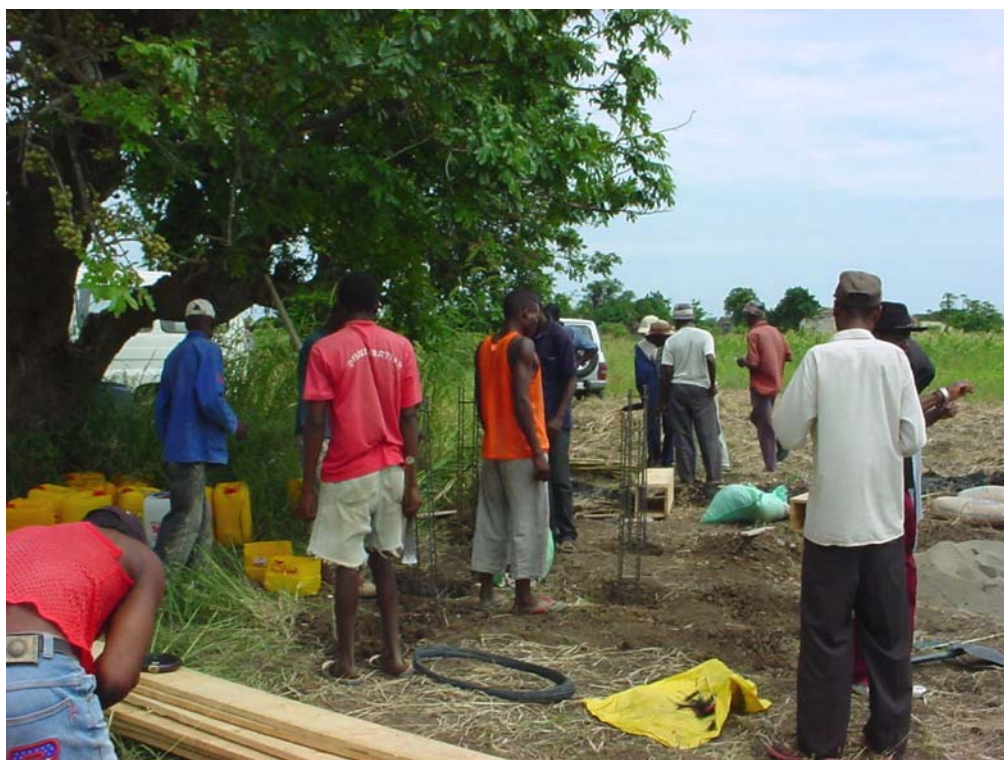
Figure 5.2 Construction of columns for rainfall harvesting facility
