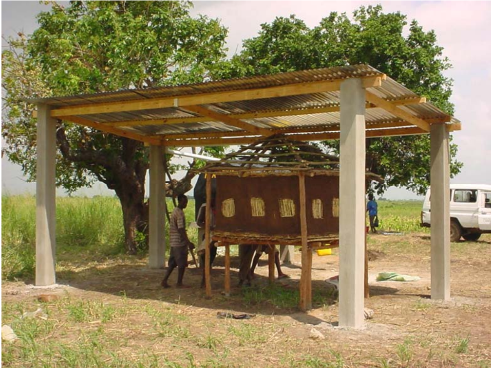
Figure 5.5 Construction of seed store
