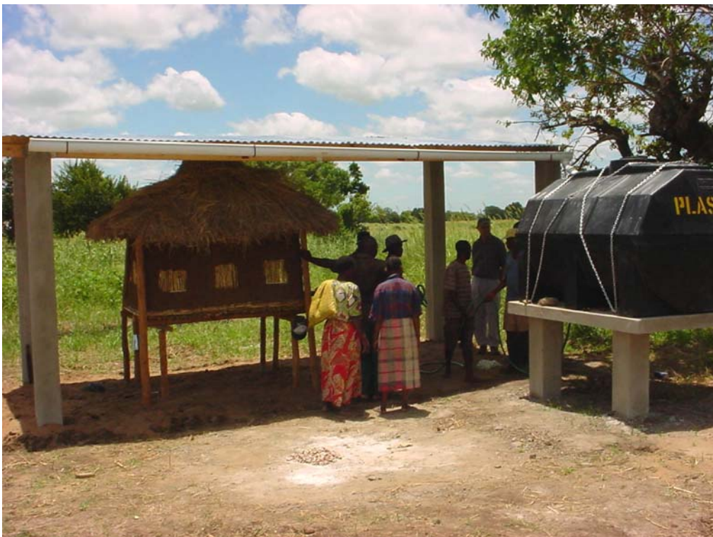
Figure 5.6 Completed rainfall harvesting facility and seed store
