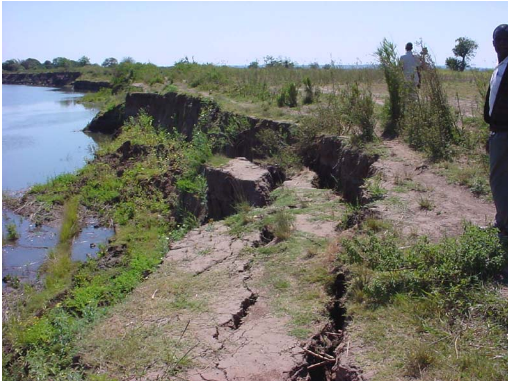
Figure 2.4 Bank erosion on the Limpopo near Languene
