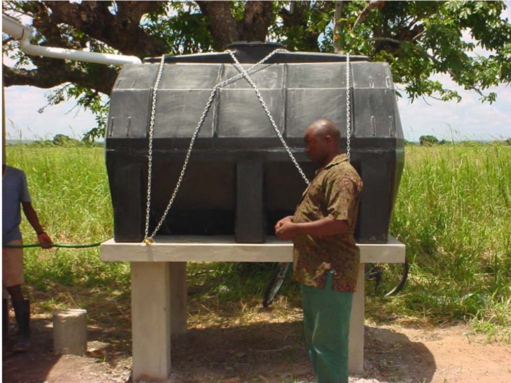
Figure 5.7 Completed water tank
