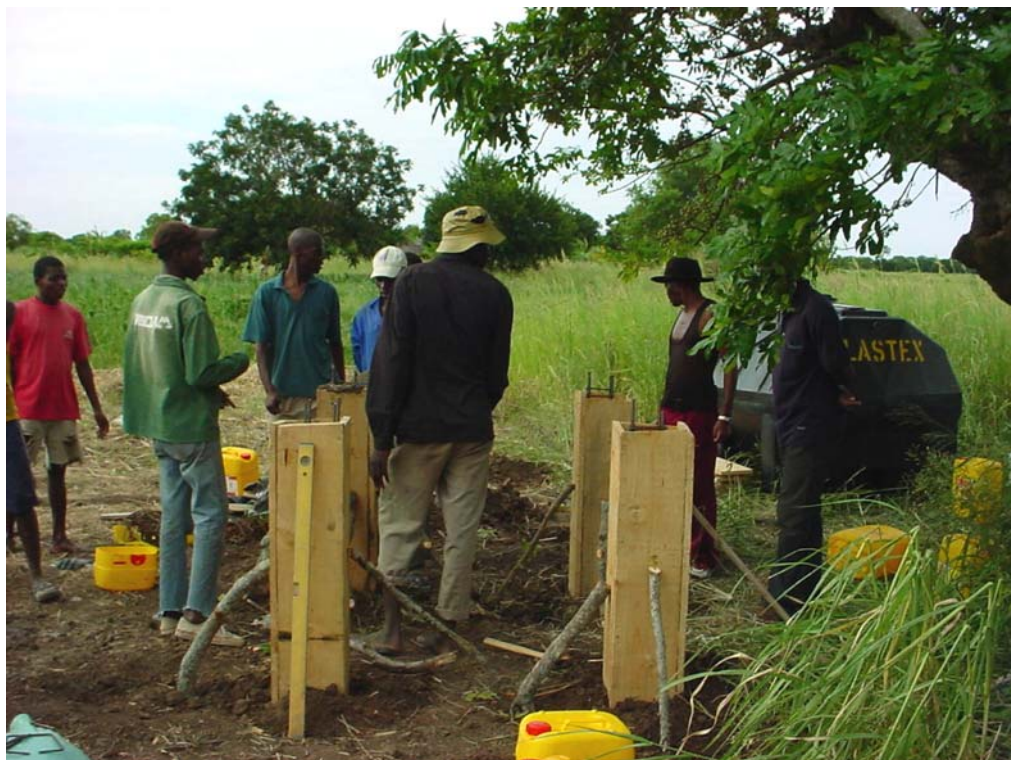
Figure 5.3 Construction of columns for rainfall harvesting facility
