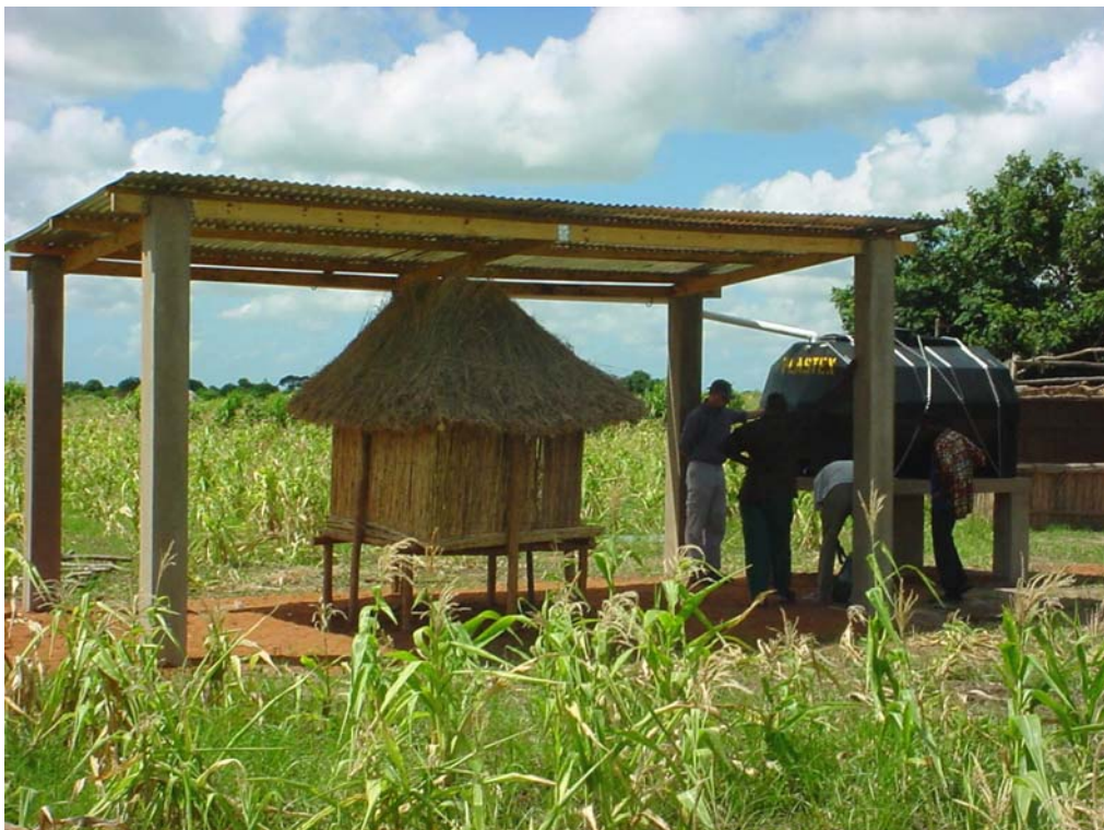
Figure 5.7 Completed rainfall harvesting facility and seed store
