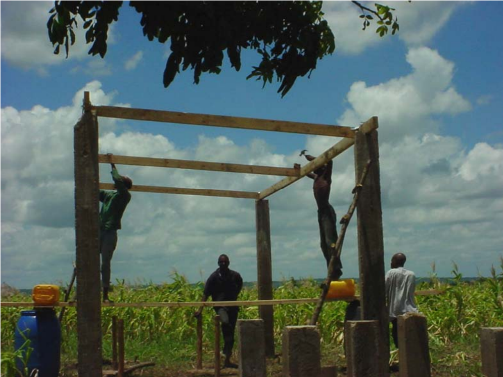
Figure 5.4 Construction of frame for rainfall harvesting facility
