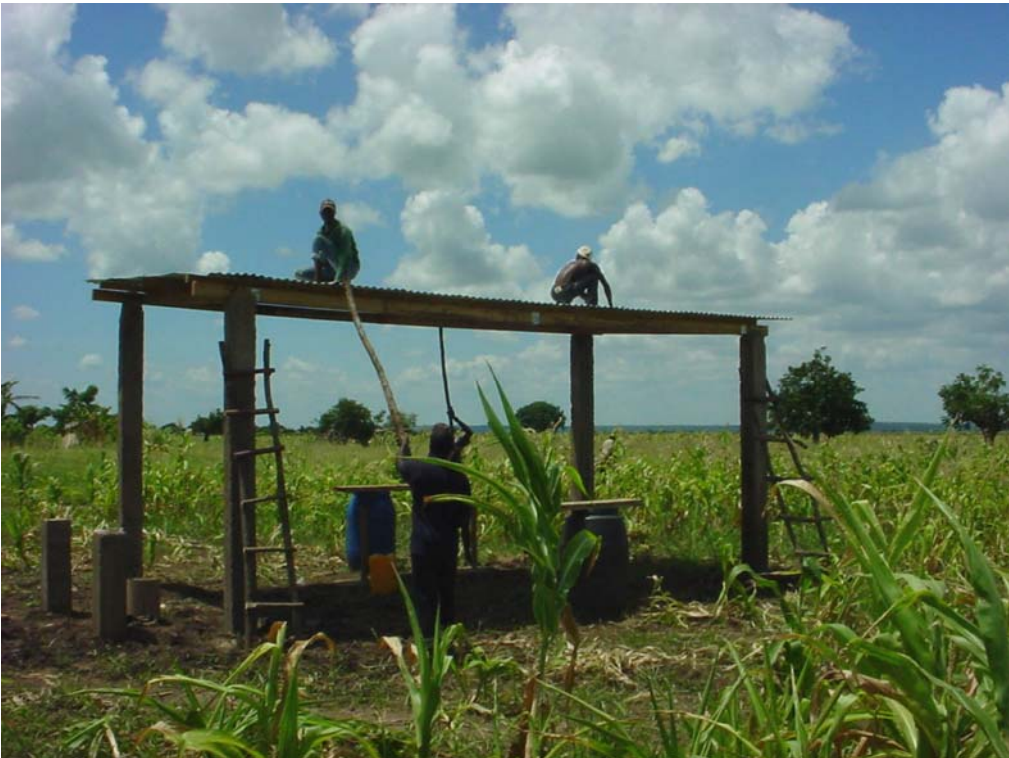
Figure 5.5 Construction of rainfall collection area for rainfall harvesting facility
