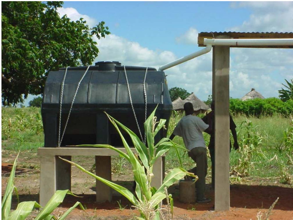
Figure 5.8 Completed water tank
