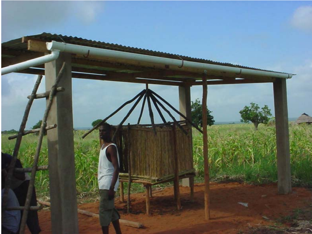
Figure 5.6 Construction of seed store
