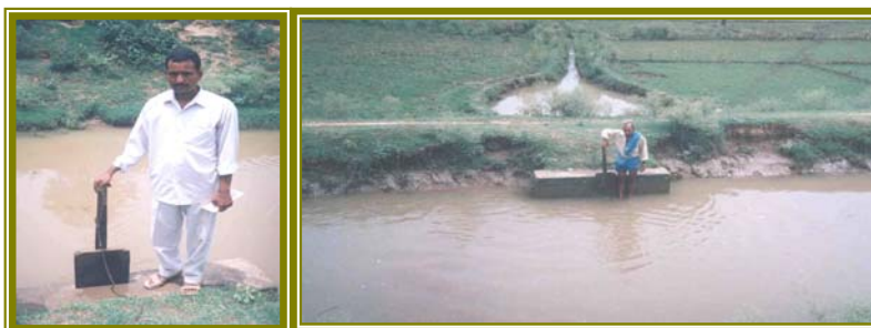
Fig – 3: Low Cost Wooden Gates fabricated and installed by OMGs
