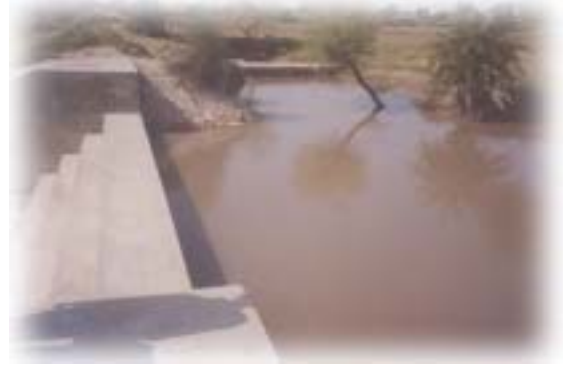
Construction of Anicuts
