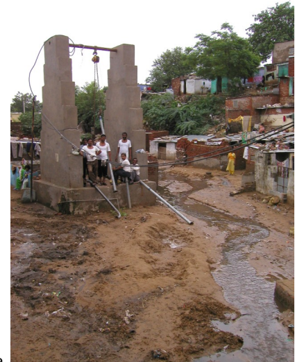
Above: Borewell maintenance
