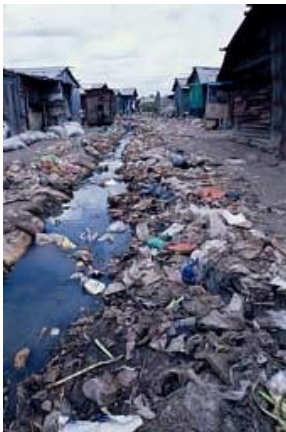
Drainage channel In Nairobi, Kenya.
