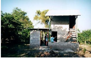
Example of a flood proof buildings in the Lempa River basin in Central America.
