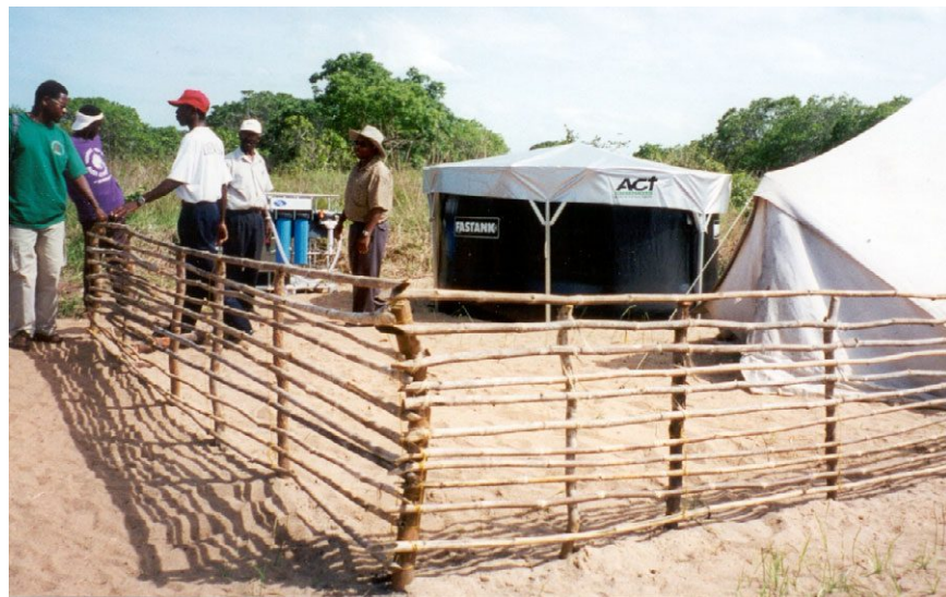
Figure 4.12 Water purification unit in Sofala Province, near Beira, Mozambique
