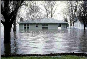
Flooded house in the USA.
