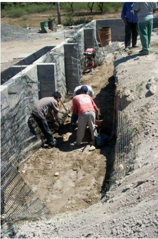
Reconstruction of houses in El Salvador after hurricane Mitch.
