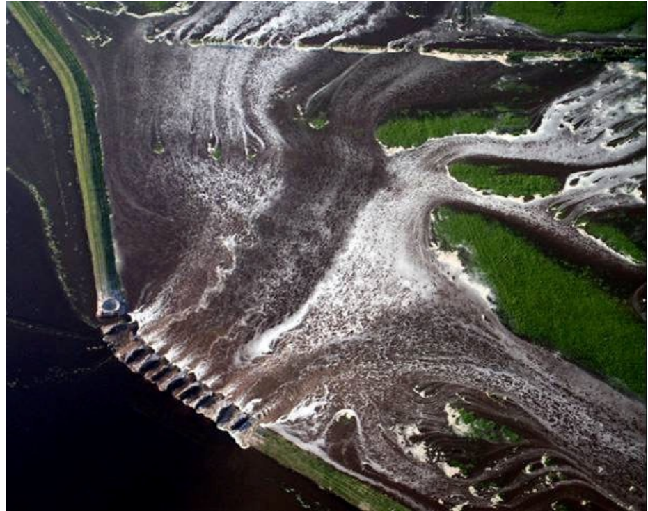
Figure 4.2 Sacrificial embankment on the River Elbe in Germany
