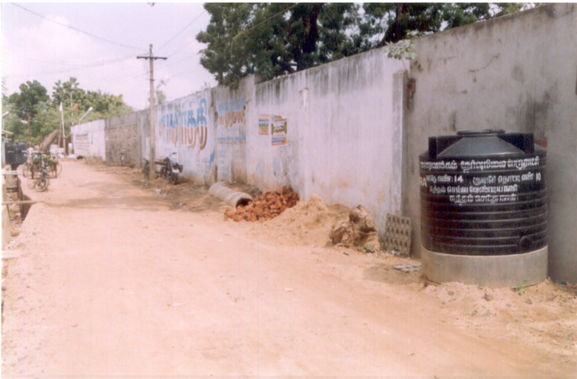
Valasaravakkam Group – Typical Sintex Tank
