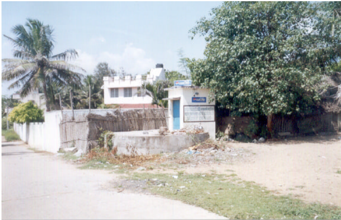
Kottivakkam Group – Typical Well & Pump Room
