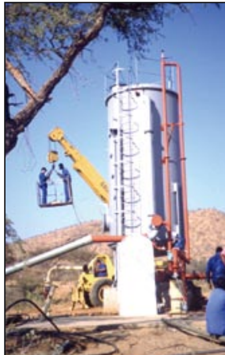
Erecting a granular activated carbon filter next to an injection borehole , Windhoek, Namibia.
