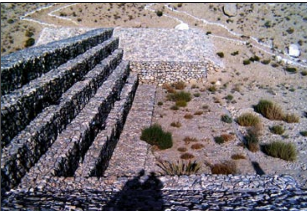
Leaky Dam Balochistan, downstream
