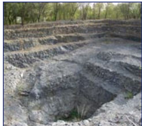
Recharge pit constructed for recharge of surface runoff, Rajasthan, India
