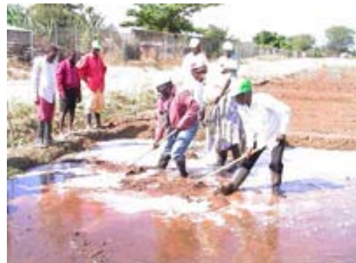
Leveling using water and simple farm tools
