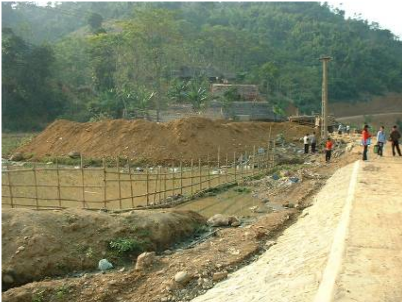
Picture 4.1: Local people show the research team an unstable section of a WB financed road where a culvert should have been built (Phu Tho)
