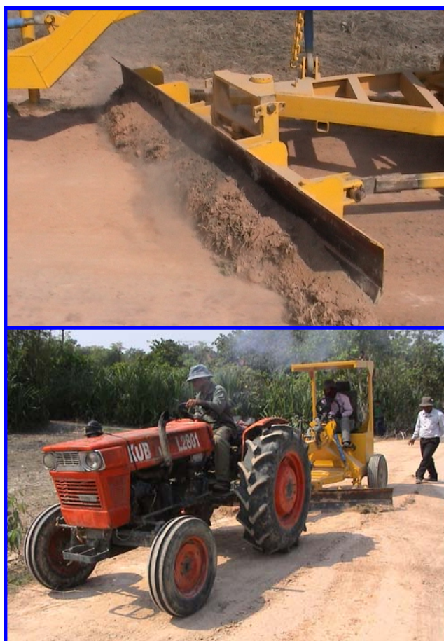
Figure 2 - ENGINEERED NATURAL SURFACES: Maintainable using simple locally made equipment & basic agricultural tractors
