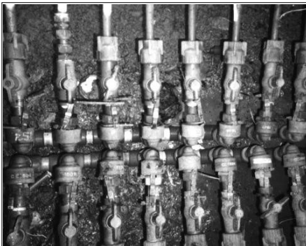
'Durban Tank': Manifold for daily household tank filling IMO Working Group, WSSCC, Kayaga Photos ↕
