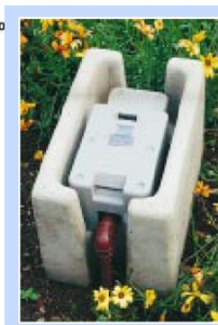
YARD METER ABOVE GROUND
