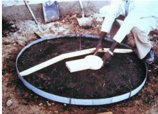
Making pit latrine slabs, Juba, Sudan
