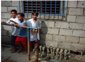
Meters replacing hand-pump, Manila, Philippines
