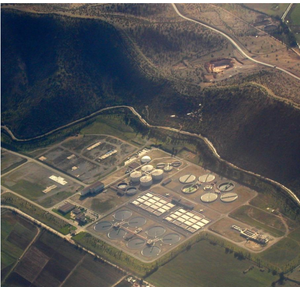
Above: New waste water treatment plant, Santiago
