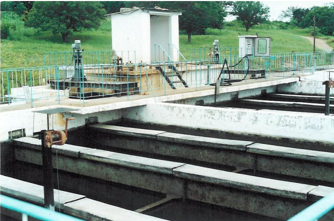
Treatment works, Zambia (NWASCO photo)
