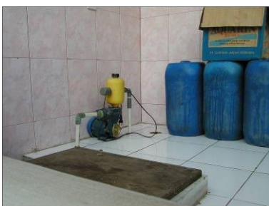
Above: household storage & pumps—low-income housing, Jakarta 18 - 8
