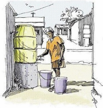
Figure 3.5. Individual yard connection with ground tank
