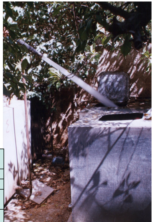
Below: Storage tank filling; note the high risk of contamination as dust and dead leaves are swept into the tank
