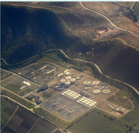
Above: New waste water treatment plant, Santiago
