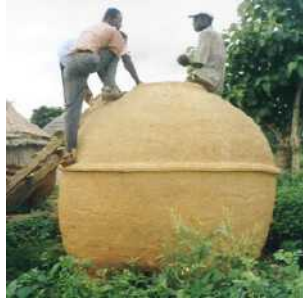
Figure 15 Mud silo at Gushiegu/Karaga with wide opening making protection from rain more difficult. The two mud silos here have collapsed on their small legs.
