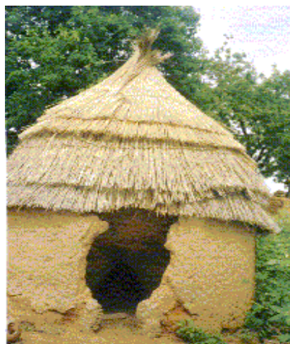
Figure 17 A mud silo standing inside a roofed fence house for protection against rains in Saboba-Chreponi district. Farmers in the newly introduced areas could be directed to do the same.
