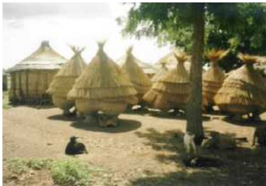
Figure 14 Thin legs of Gushiegu/Karaga mud silos, set on rounded instead of flat stones
