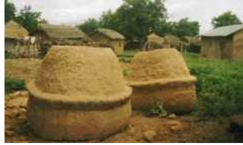
Figure 16 A Kokomba mud silo tapered into a small opening at the top making coverage easier.
