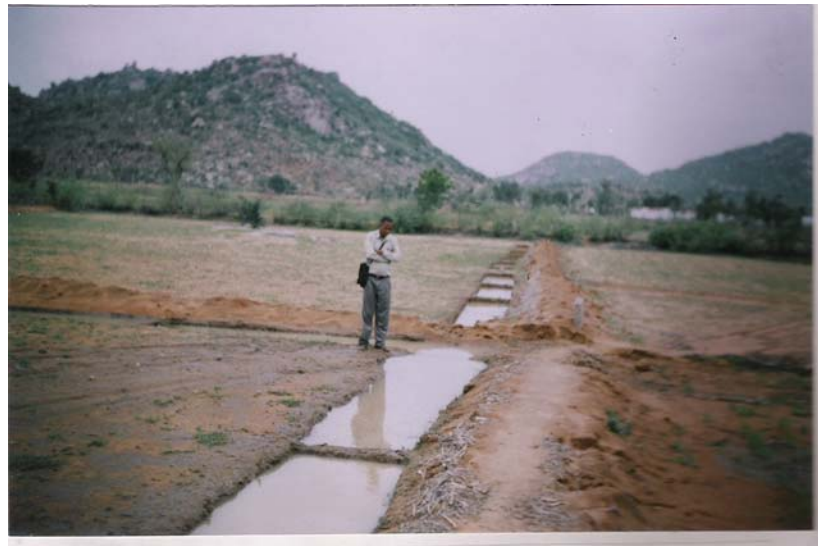
Trench cum bund for conservation of soil & water in M'nagar
