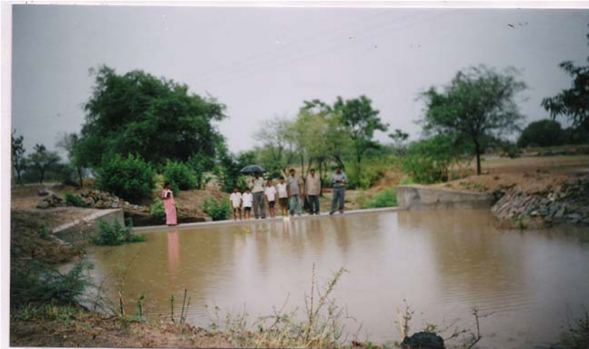
Check dam filled to brim during first rain in M'nagar
