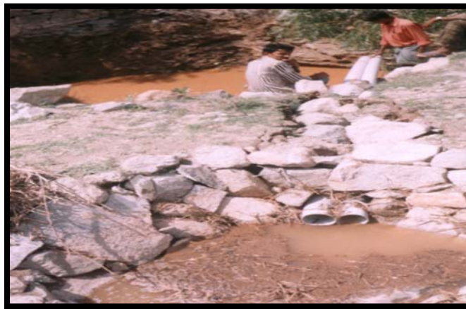
Recharging defunct wells through rain water diversion in A'pur
