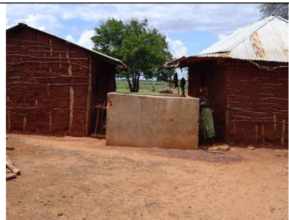
Plate 4: Roof-top RWH with a storage structure in Bangalala village
