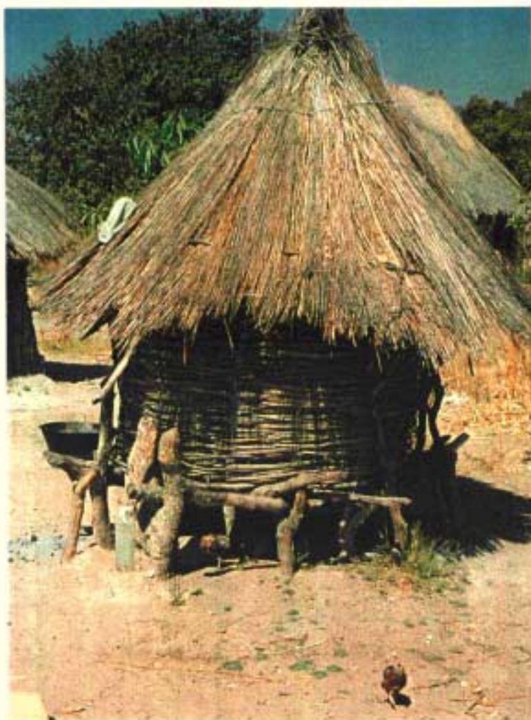
Typical mud and basket storage structures found in the region
