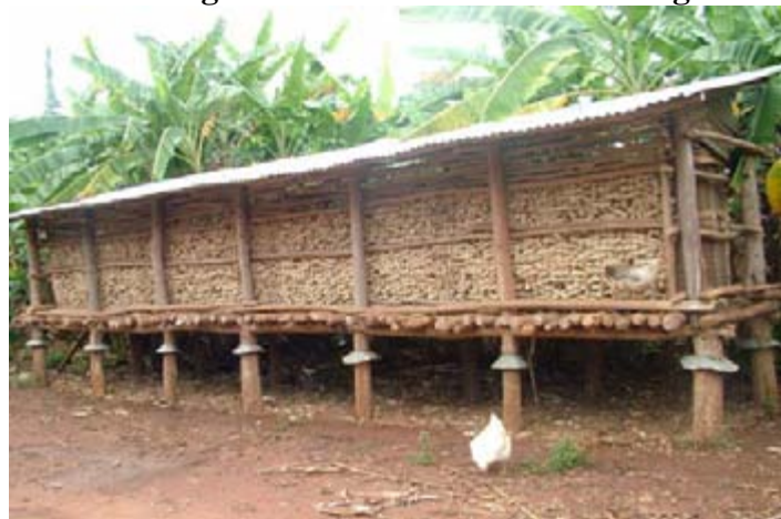
Fig 16. Improved crib used to store maize in Iganga district
